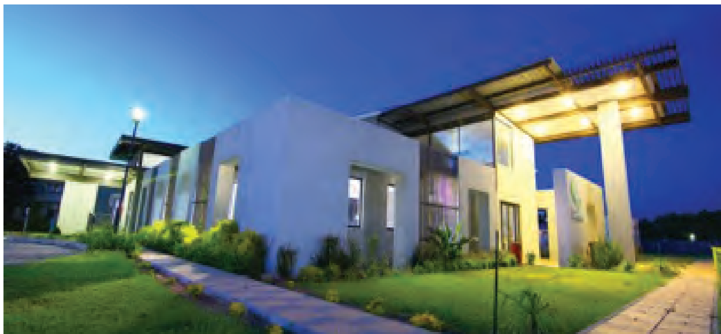
Figure 3: Entrance/drop off area
